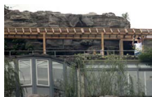
Demolition work starts on rooftop villa structure
